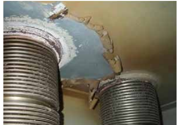
External Penetration Hot Spot
