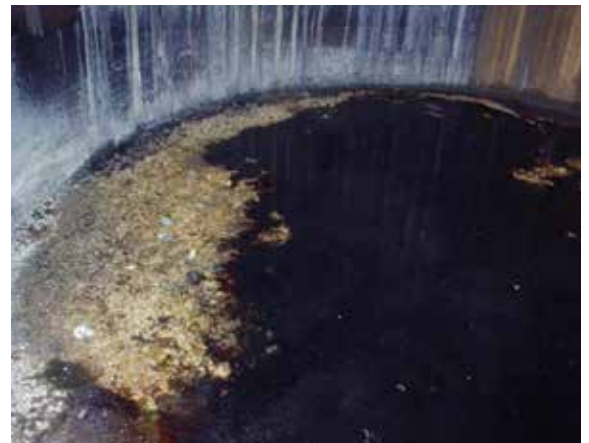
Stack Corrosion
