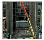
In cases where site access is limited, Vogt Power will reduce the pre-assembly and supply a V-Lite design. Individual module harps are transported to the site using normal road transportation.
