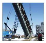
Semi-Modular Accelerated Delivery Reduced Cost Top Supported is used when shipping constraints prevent the use of the V-Max design. Our V-Flex design is highly pre-assembled; modules, casing, interconnecting piping, and some of the structural steel are all contained in each module box.
