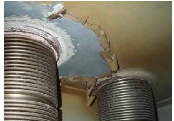
Inspection of External Penetration Hot Spot
