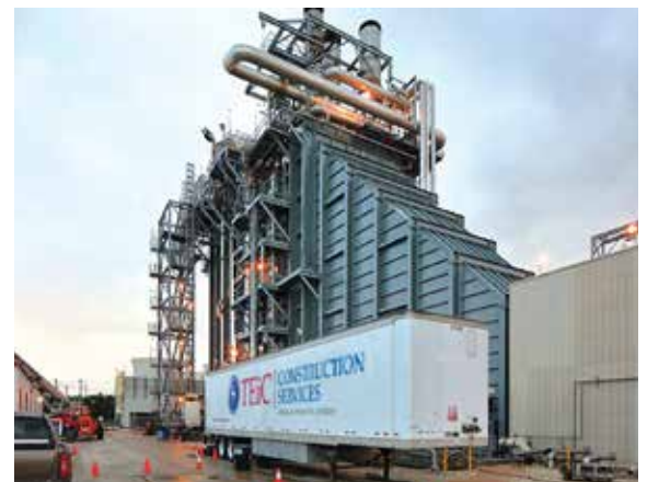
TEiC on site of HARP retrofit
