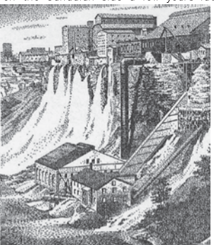
Produced the first penstock on the American side of Niagara Falls and the first on the Canadian side a few years later.
