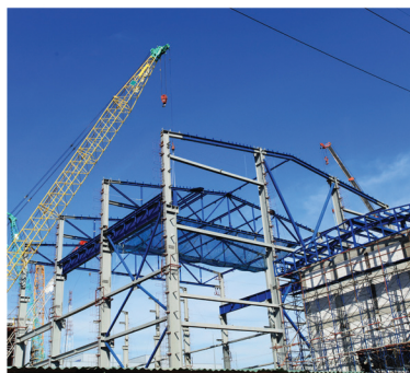
Building Structural Steel Erection
