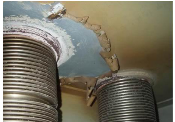
Inspection of External Penetration Hot Spot
