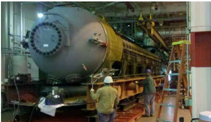
Bundle replacements are just one of many retrofit solutions
