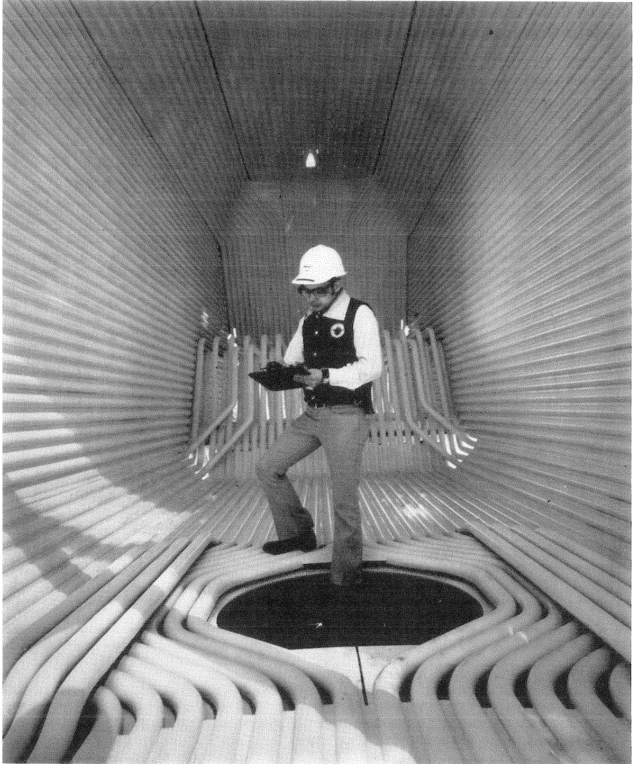
Figure 9 Internal View of Furnace Module and Boiler Opening
