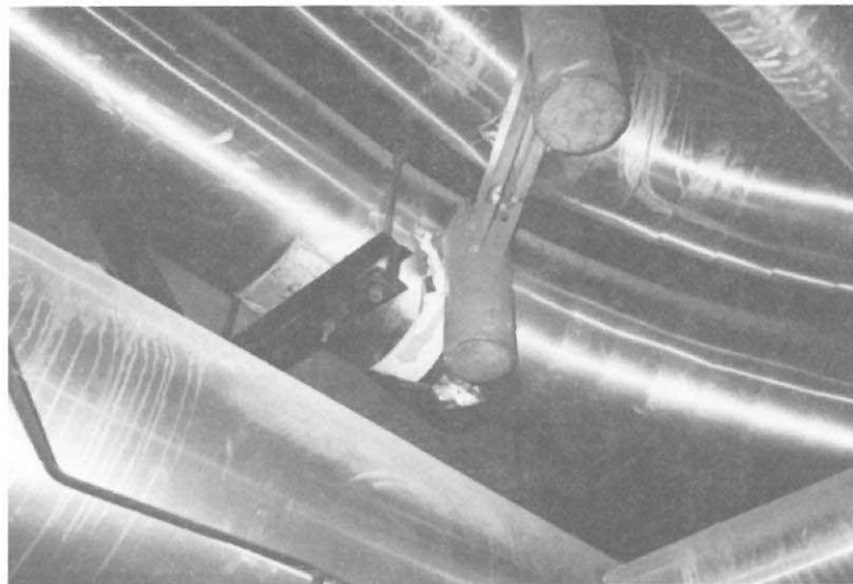
Figure 4 (top) and Figure 5 (bottom) - Case No. 2 Main steam piping constant force support assembly, which appear to be slightly tilted to one side. Also, the parallel supports show different position indications in the cold condition.
