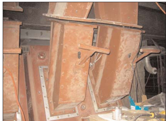
Figure 6. Coal Head with Turning Vanes
