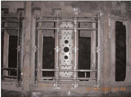
Figure 3. Perforated Plate and Air Chamber
