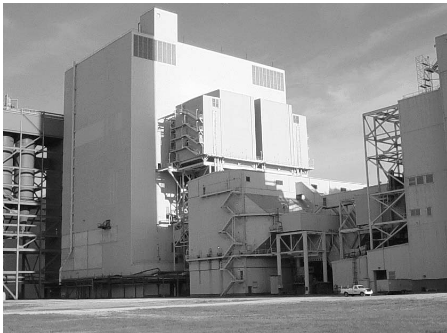
Figure 3 Trimble County completed SCR retrofit
