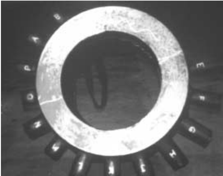
Figure 3 Sample Piece of Radiant Superheater Outlet Header
