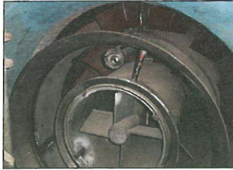
Figure 4. RPI CCV DAZ Burner Installed in 500 MW Utility Boiler
