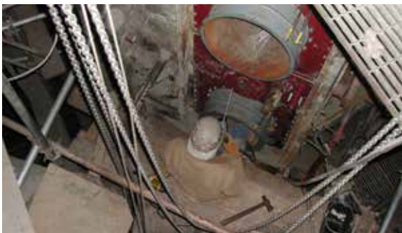
Corner Fired Burner Replacement
