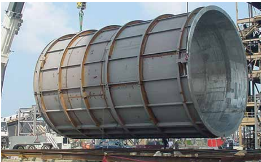
Erecting Scrubber (FGD)
