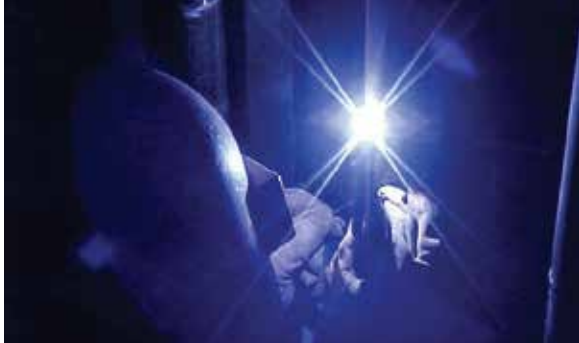
Boiler Tube Welding
