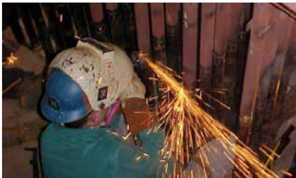
Boiler Super Heat Replacement
