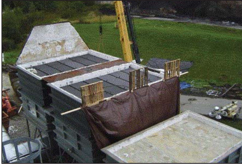
Figure 10. A 3-Canister system under construction.
