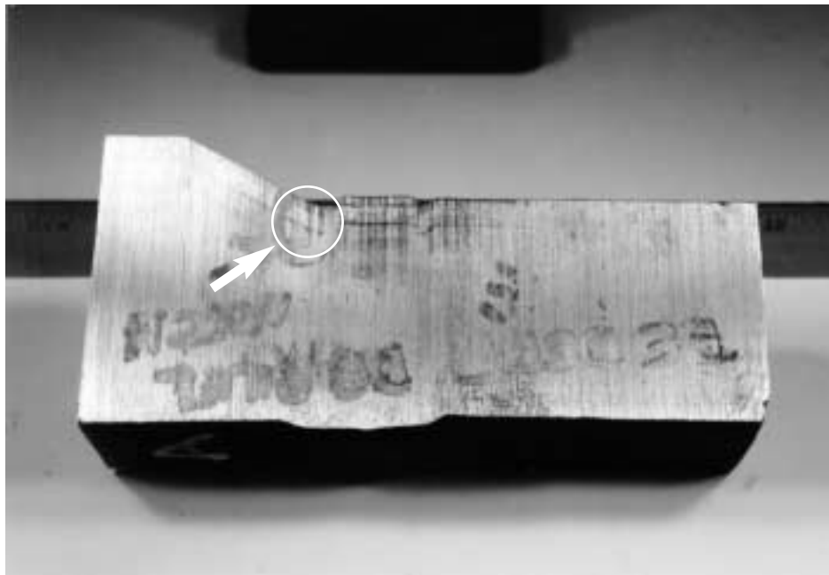
Figure 6 View of the cut cross sectioned surface showing the location of the crack at the taper transition at the ID of the elbow
