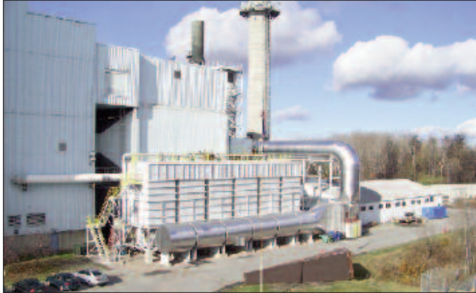
Figure 6. An RSCR system with six canisters on a 50 MW unit
