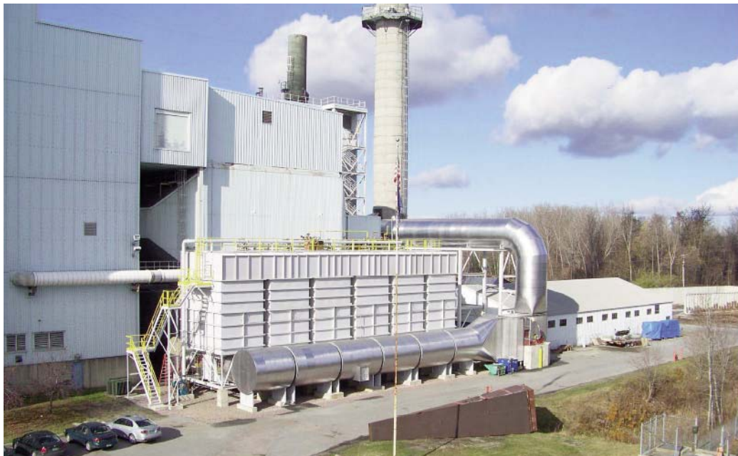
An RSCR system with six canisters on a 50 MW unit
