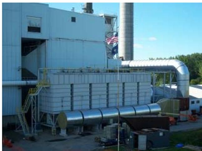
Figure 7: An RSCR system with six canisters on a 50 MW unit.
