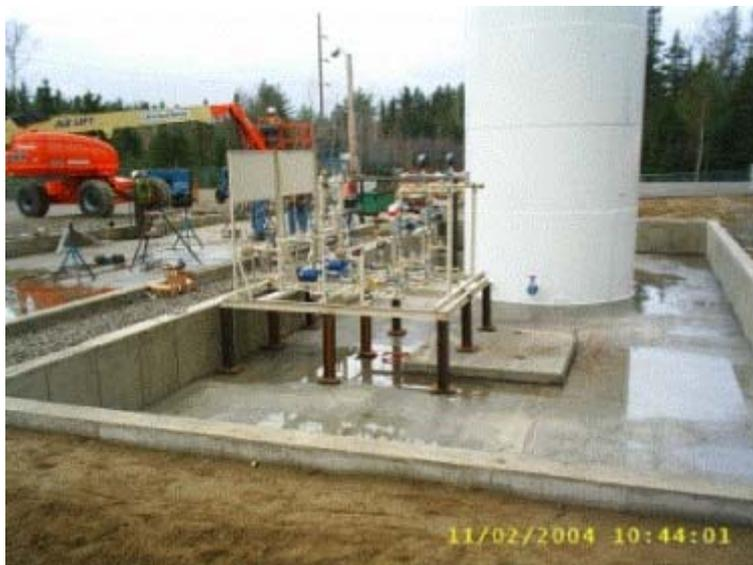
Figure 5: Ammonia skid/storage tank -50 MW RSCR.
