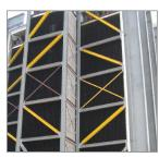
For HRSGs where transport and weight limitations allow, the main steel support structure is integrated and pre-fabricated with the boxes in a design that is the ultimate in constructability.
