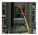
In cases where site access is limited, Vogt Power will reduce the pre-assembly and supply a Loose HARP design. Individual module harps are transported to the site using normal road transportation.
