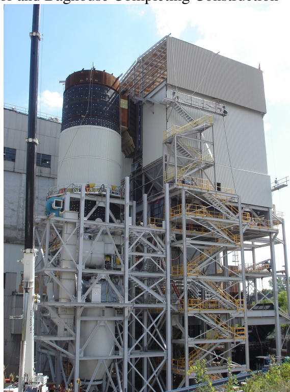
Figure 6 Turbosorp Reactor and Baghouse Completing Construction
