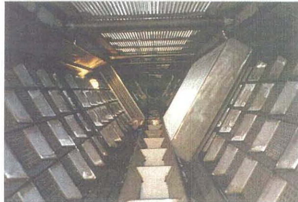
MOISTURE SEPARATION SECTION - INSTALLATION Figure 2
