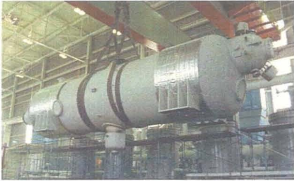
A NEW MSR VESSEL - INSTALLATION Figure 9
