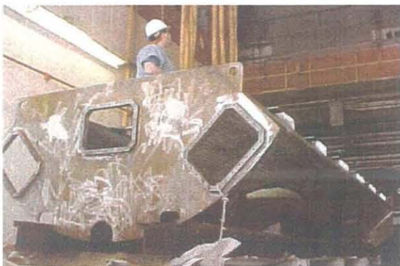
MOISTURE SEPARATION MODULE INSERTION Figure 13
