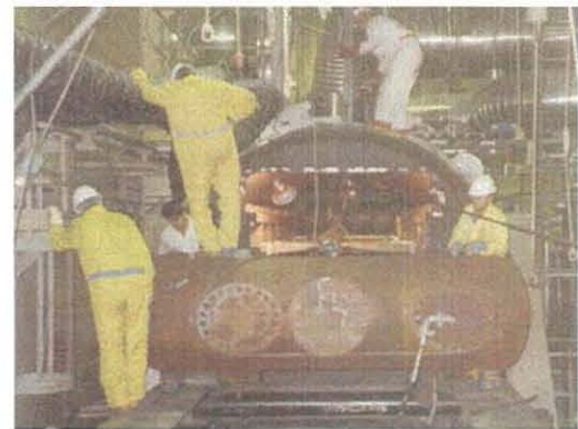
REHEATER INSTALLATION - ACTUAL Figure 12b
