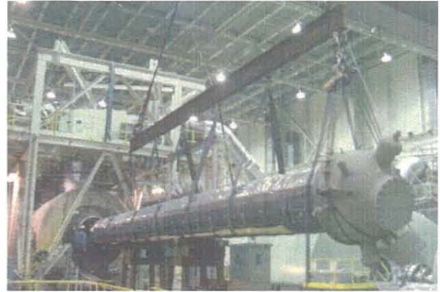
REPLACEMENT REHEATER - INSTALLATION Figure 10
