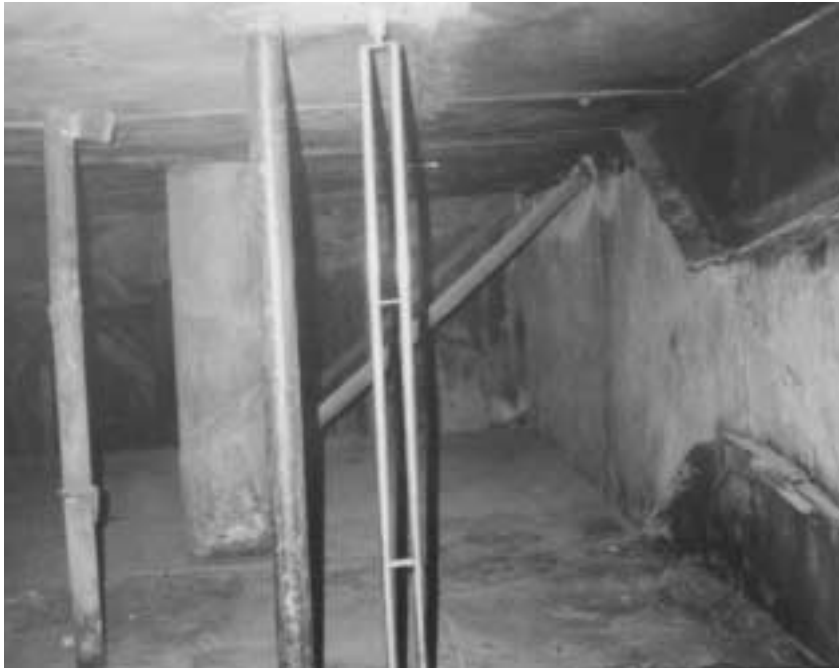
Figure 11 Secondary Air Flow Measurement
