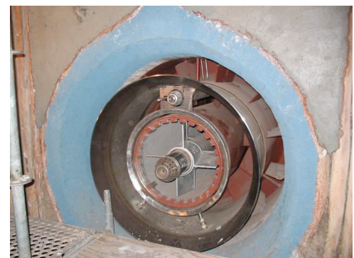
Figure 10 VS III™ Burner Installation w/Igniter in SA Annulus
