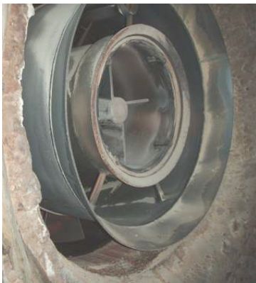
Figure 7 210 mmBtu/hr capacity burner on Foster Wheeler unit after 2 ½ years of operation (medium abrasive Galatia Bituminous coal)
