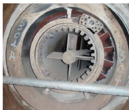
Figure 9 150 mmBtu/hr capacity burner after 3 years of operation on PRB Coal - 750 MW Opposed fired boiler
