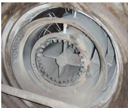
Figure 9 150 mmBtu/hr capacity burner after 3 years of operation on PRB Coal - 750 MW Opposed fired boiler
