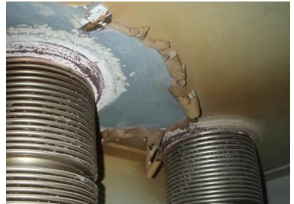
External Penetration Hot Spot
