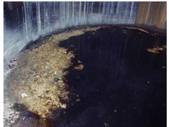
Stack Corrosion
