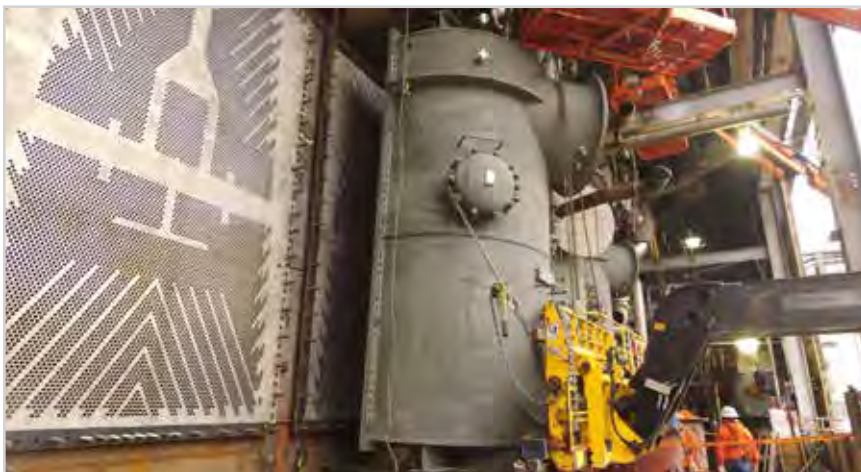
Steam Surface Condenser Modular Changeout
