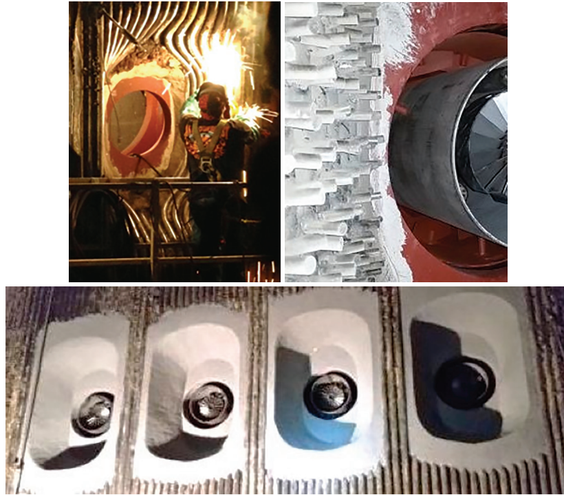
Figure 8 — Unit 10 Burner Throat Refractory Installation
