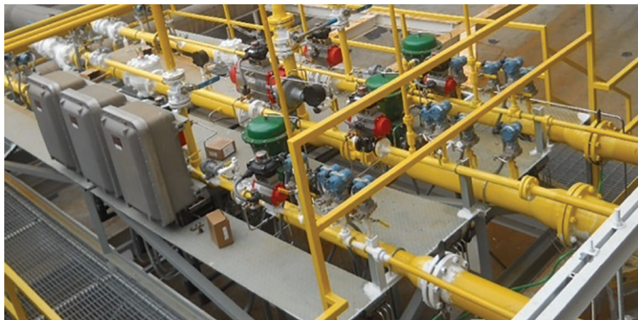
Figure 4 – Natural Gas Control Skid, all three (3) Boilers
