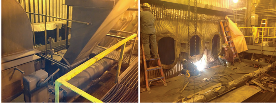
Figure 6 – Unit 10 Existing Bark Feed Chute and Nozzle (left), and Bark Feed Openings after Demo (right)
