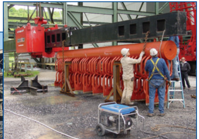
REPLACING MAIN STEAM OUTLET HDR
