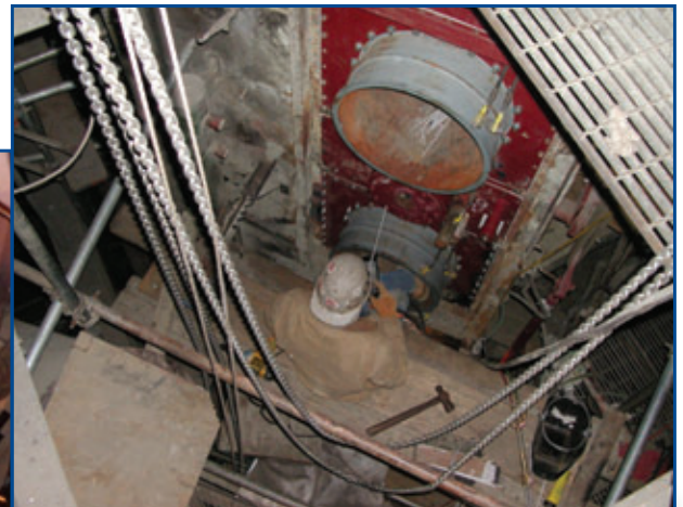
CORNER FIRED BURNER REPLACEMENT
