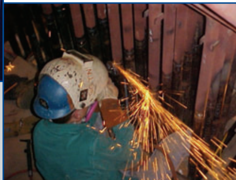
BOILER SUPER HEAT REPLACEMENT
