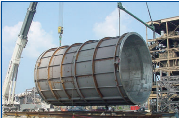
ERECTING SCRUBBER (FGD)
