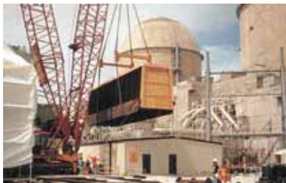
Condenser Modules being picked up by crane in preparation for installation
