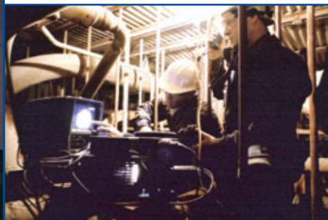
FIBEROPTIC IMAGING USED FOR INTERNAL INSPECTIONS
