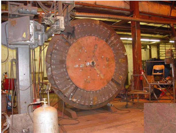
Pulverizer Bull Ring Segments setup on fixture ready for grooving.
