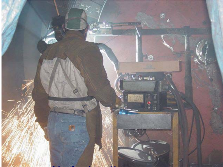
Air Arcing the grooves in Bull Ring Segments
